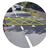
Raised pedestrian crossing
